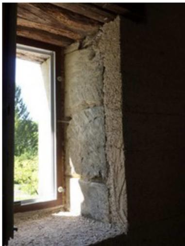
Figure 2-5 : Mortier chaux-chanvre sec
