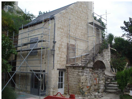
Figure 1-7 : Restauration de la façade
