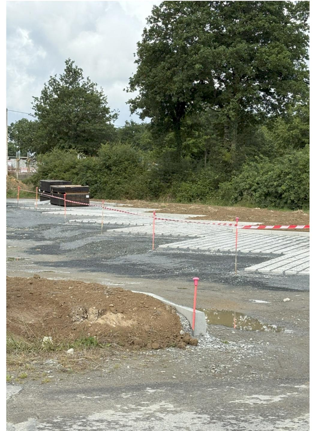
STATIONNEMENTS PAVES BÉTONS JOINTS ENHERBES
