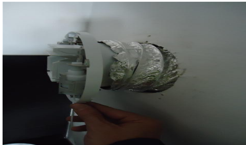
Gaine mal raccordée
