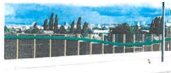
Liège - facade de Lougny - Architecture : Sobotta
