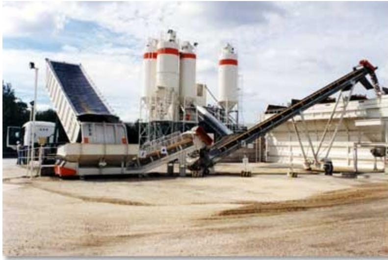
Illustration 1: Centrale à béton - photo UNICEM
